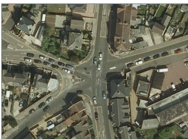
Figure 18 – Victoria Traffic Signals
